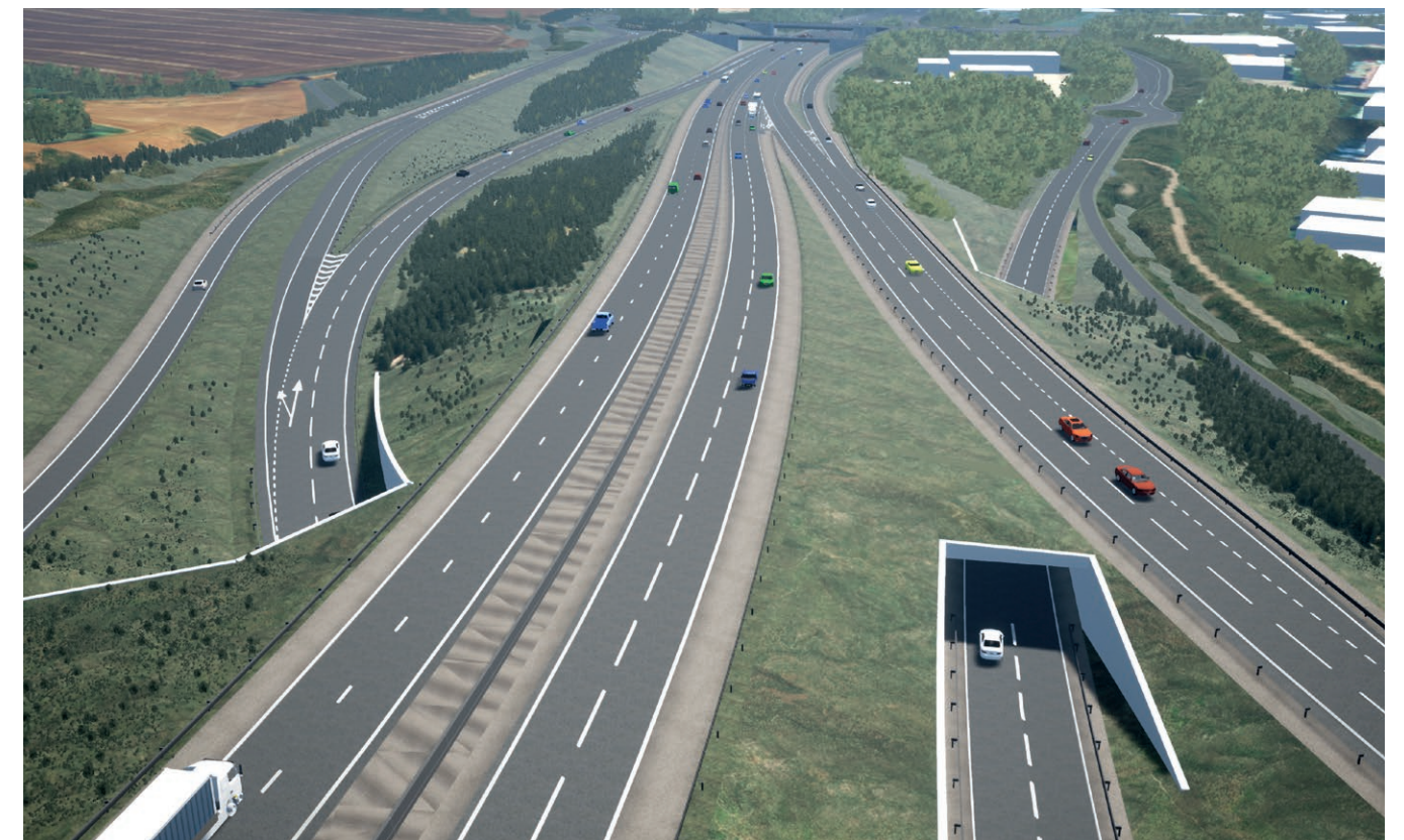
New A34 (left) and A33 (right) underpasses - M3 southbound
