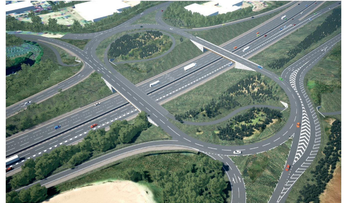
New junction 9 roundabout
